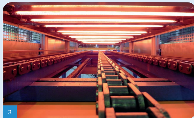
3 Inside the Infrared Oven.
