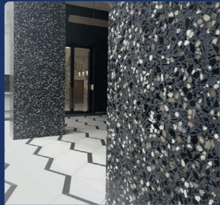
Wall-cladding tiles: low relative weight and high compactness of the tiles produced allow use for exterior cladding of buildings and industrial units.
